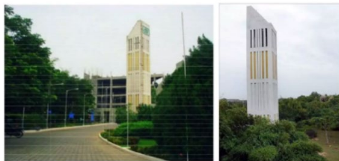
Figure 24 Showing the Wind Catcher as an Element for Natural Ventilation
