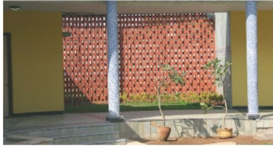
Figure 19 Showing the use of Brick Jali Wall as a Façade for Natural Ventilation
