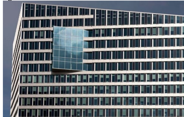
Figure 7 Exterior View Showing the Arrangement of Solar Panel and Glass as a Grid
