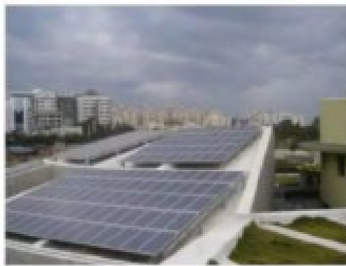
Figure 28 Showing the Application of Solar Panels on the Roof of the Building
