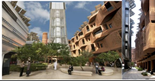
Figure 6 Masdar Wind Towers are Contemporary Adaptations of Traditional Windcatchers, Engineered to Naturally Cool Public Areas by Directing Breezes, Minimizing Energy Usage, and Improving Comfort in the Arid Atmosphere of Masdar City
